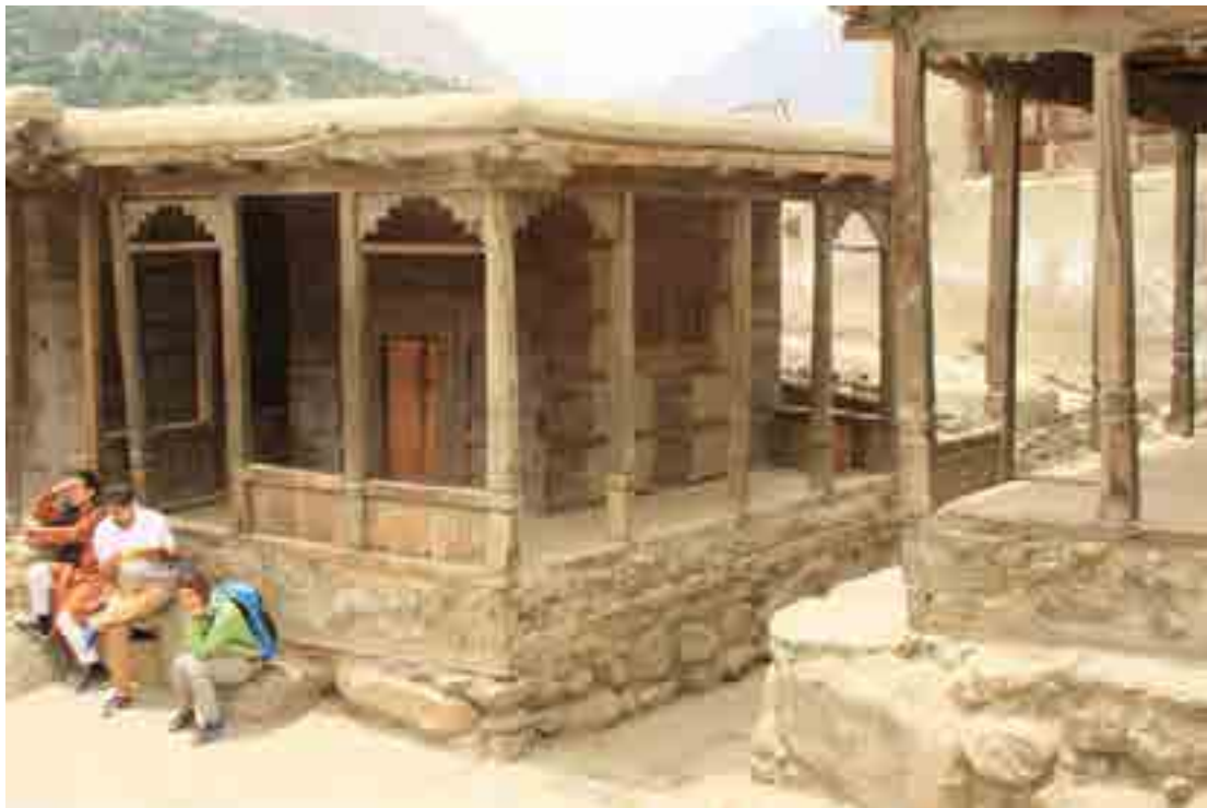
Researchers rest at the historic timber construction mosques of Ganish Settlement, Hunza Valley, Pakistan.
