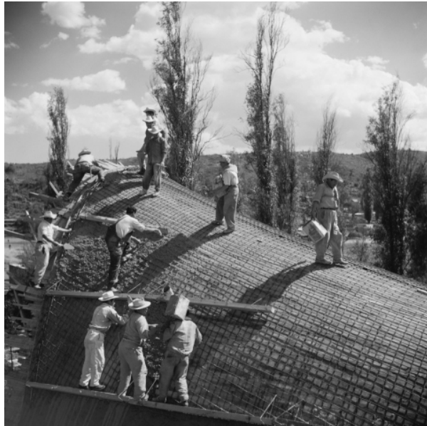
Workers constructing the concrete shell at Restaurante Los Manantiales in Xochimilco, Mexico City in 1958
